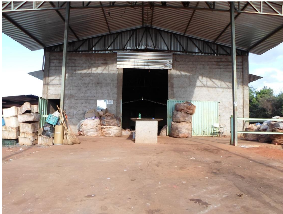
Figura 7.166 – Entrada principal da UTC Papagaios
